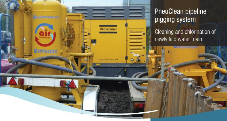
HTC, part of the Aquam group, has undertaken cleaning and chlorination of a newly laid water main that runs underneath the A1, the UK's longest road. Contractor Balfour Beatty selected Aquam's PneucleanTM pipeline pigging and chlorination system on behalf of Anglian Water's @One Alliance for the Kings Reach Growth Pipeline project.
